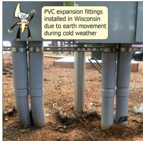
Earth movement resulting in PVC raceway being pulled loose from the male adapter
